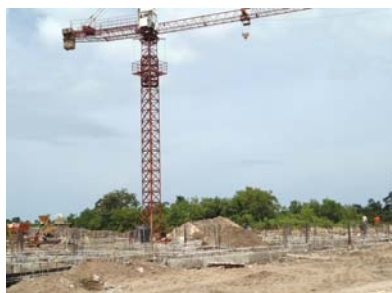
Progress on Sierra units
