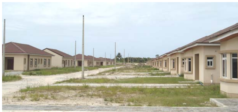
Row of finished homes with ongoing infrastructure works
