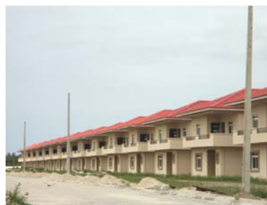
Sirocco units with electricity poles
